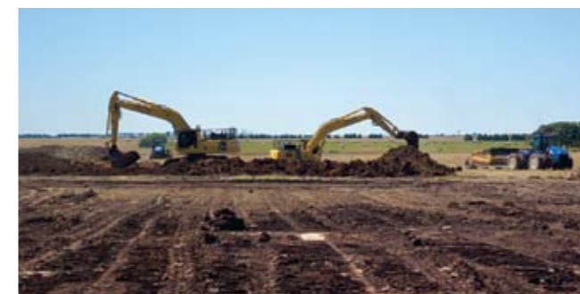
Construction of Macarthur Wind Farm is underway Source: AGL Energy
