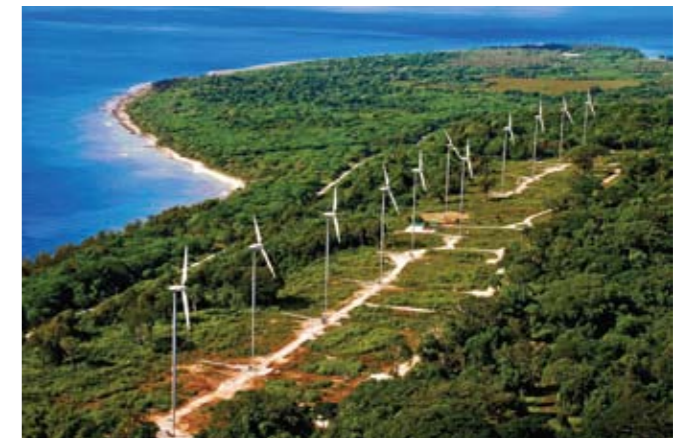
Unelco Wind Farm, Efaté, Vanuatu, comprising 11 Vergnet 275 kW turbines
