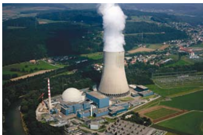
Pressurised Water Reactor, Gösgen Nuclear Power Plant, Switzerland
