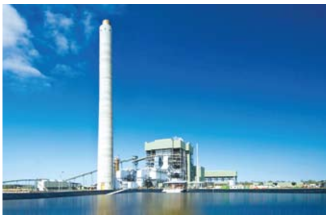
Kogan Creek Power Station
