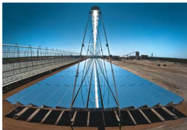
AREVA's solar CLFR technology
