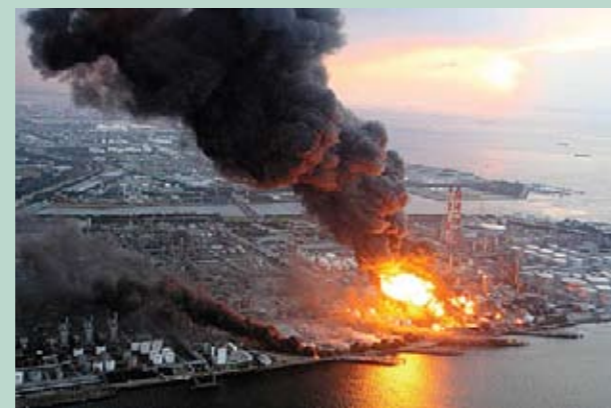
Fire at the Chiba refinery, Japan Source: Flickr
