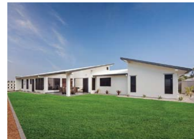
InsulLiving Home, Burpengary, Queensland
